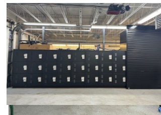
South Garage-After, FY25
