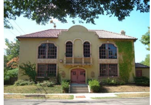
Water Pumping Station
