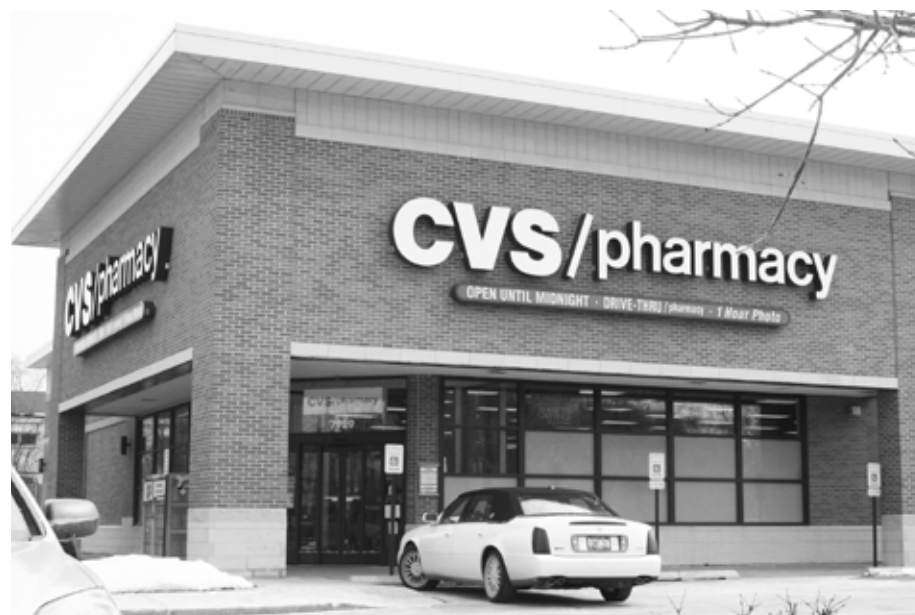
New construction in the Village at the southeast corner of North Avenue and Thatcher Avenue.
