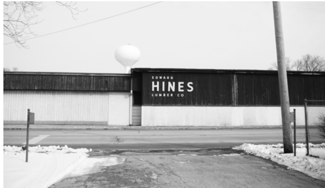
A key redevelopment site along Madison Street.
