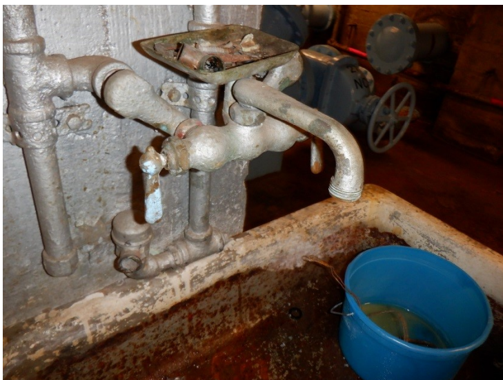
39) There is a threaded sample tap on the piping in the building.
