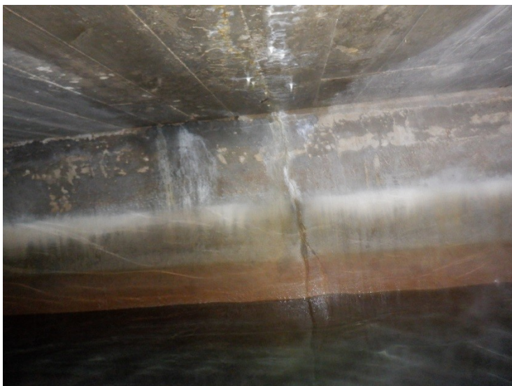
18) There are a few cracks on the wet interior concrete sidewall.
