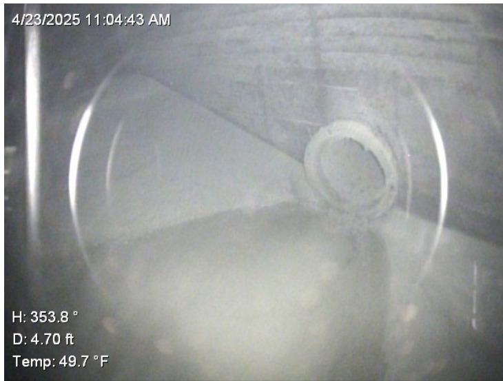
28) The draw pipe penetrates the concrete sidewall.
