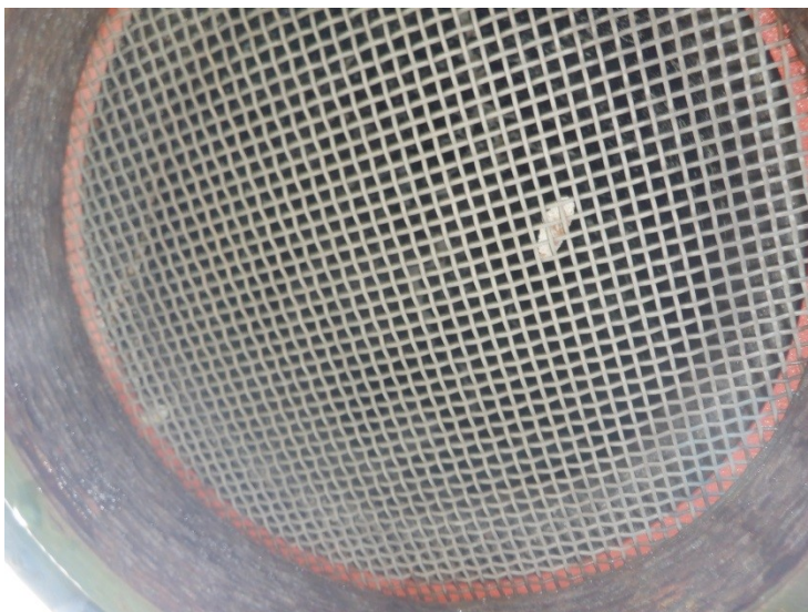
3) The goose neck vent screen is intact but oversized.
