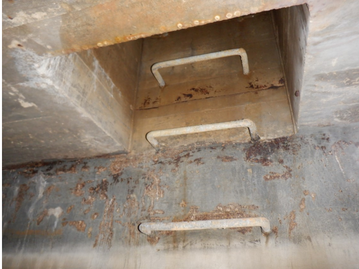
10) The wet interior ladder cleats appear to be in good condition.
