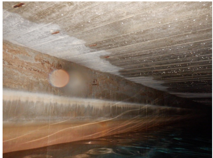
20) The wet interior concrete sidewalls are in good condition overall.
