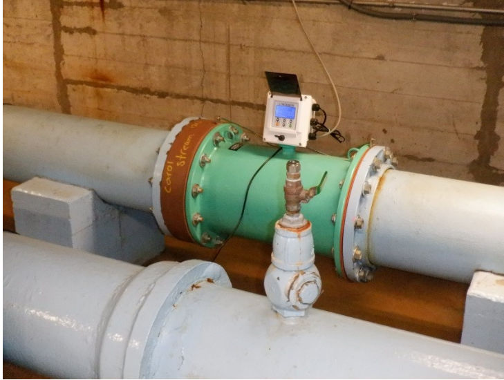
37) The pipe coating in the building is in good condition with minor surface corrosion.
