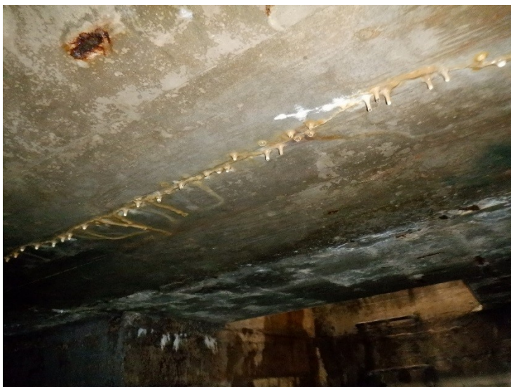
12) There are a few cracks with efflorescence present on the wet interior concrete roof.
