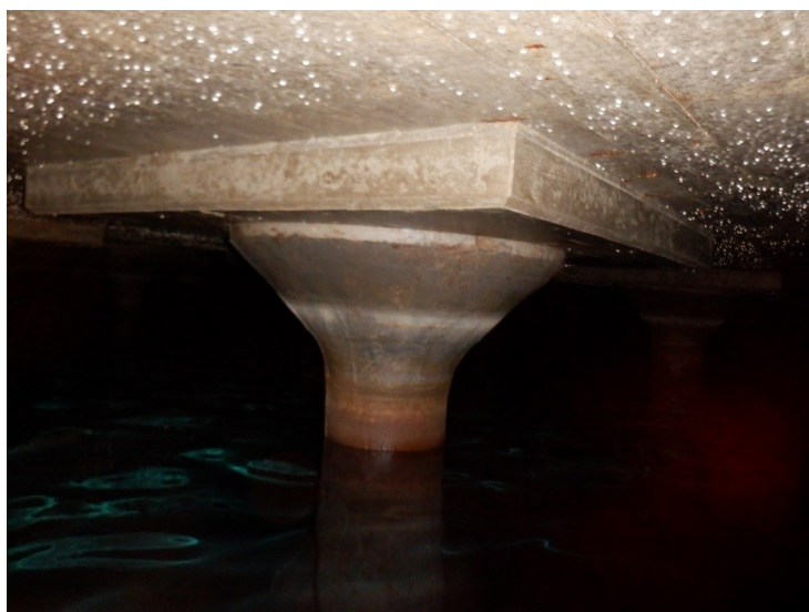
30) The concrete columns are in good condition with no deterioration.
