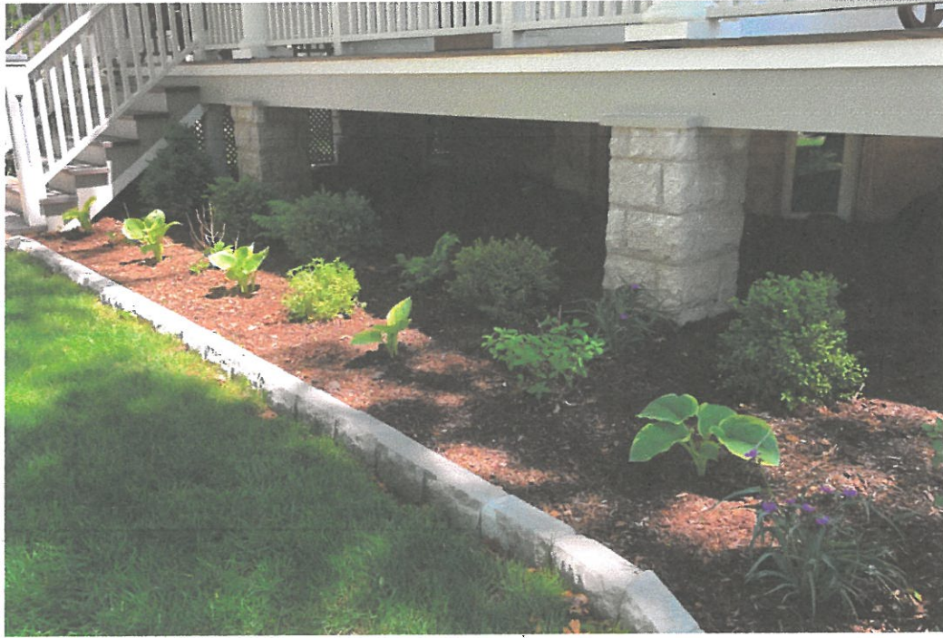
AFTER RESTORATION ( porch support matching foundation stone, side yard )
