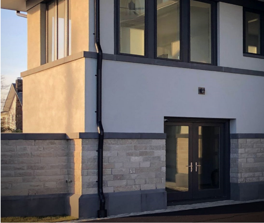
Image 1, Masonry knee wall example
