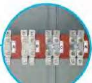
Lugs are labeled for connection sequence
