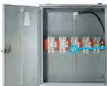
Generator lugs rated for Type VV cables
