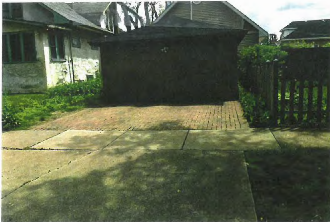
GARAGE FRONT ASHLAND AVE
