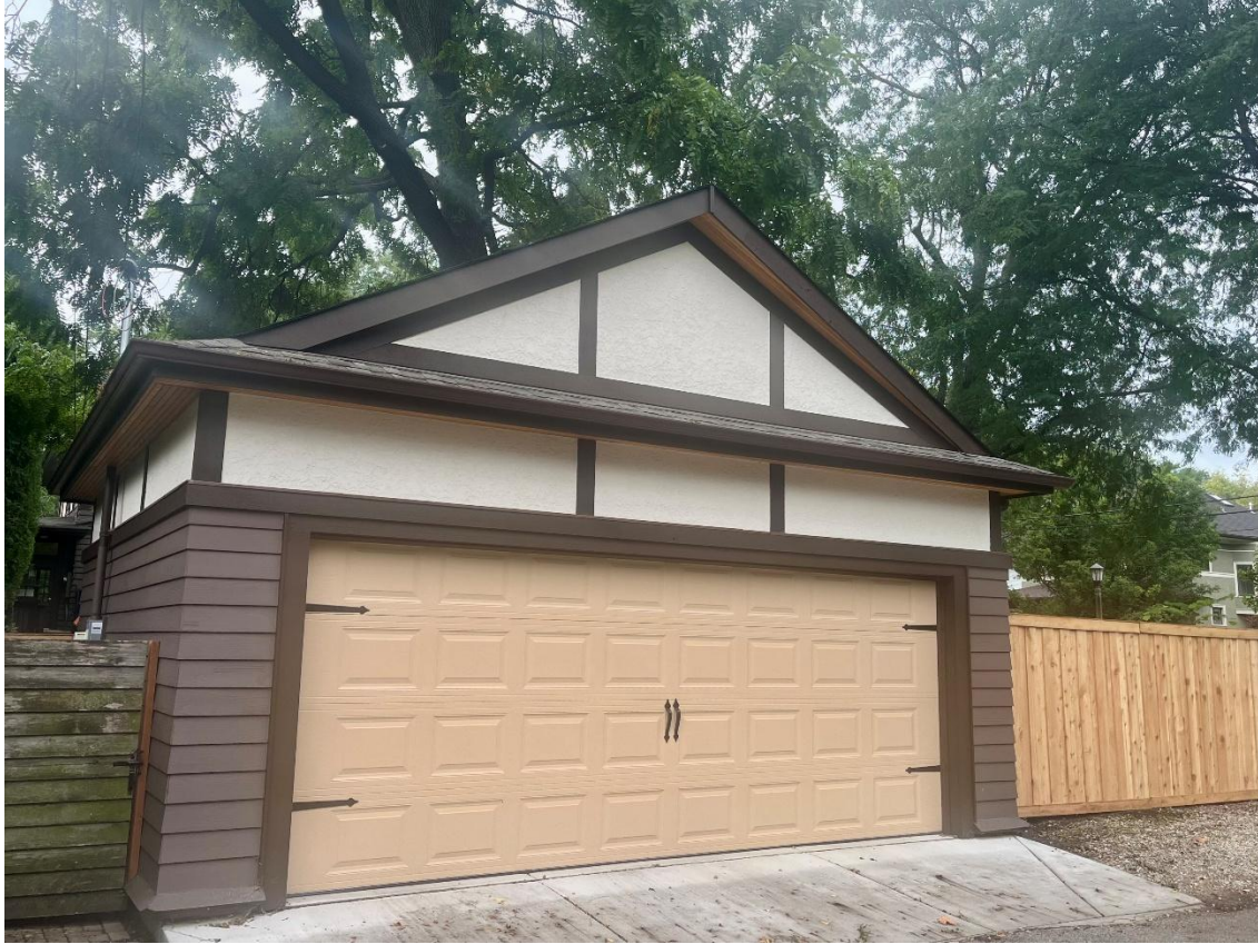
View of new garage from alley
