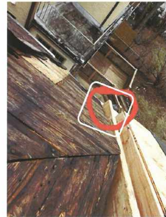
View of existing roof and new addition roof highlighting roof sag conflict
