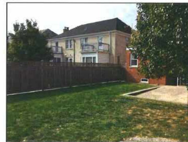
7 VIEW LOOKING SOUTHWEST
