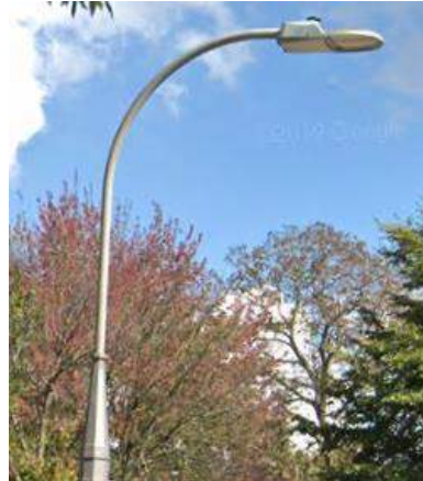
Proposed goose-neck fixture (16 ft. high):
