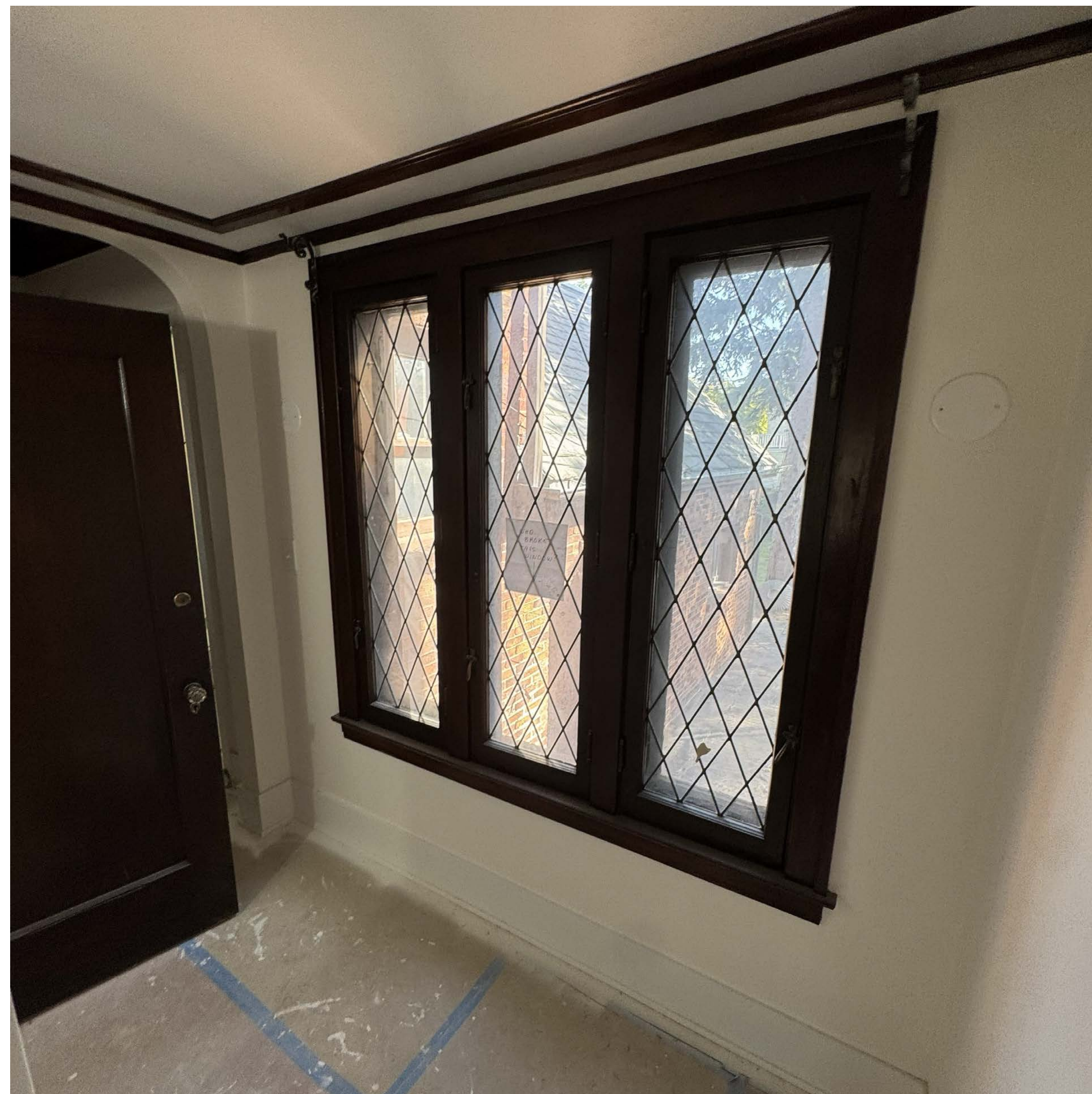
ORIGINAL LEADED GLASS WINDOW VISIBLE FROM INTERIOR (EXTERIOR STORMS)
