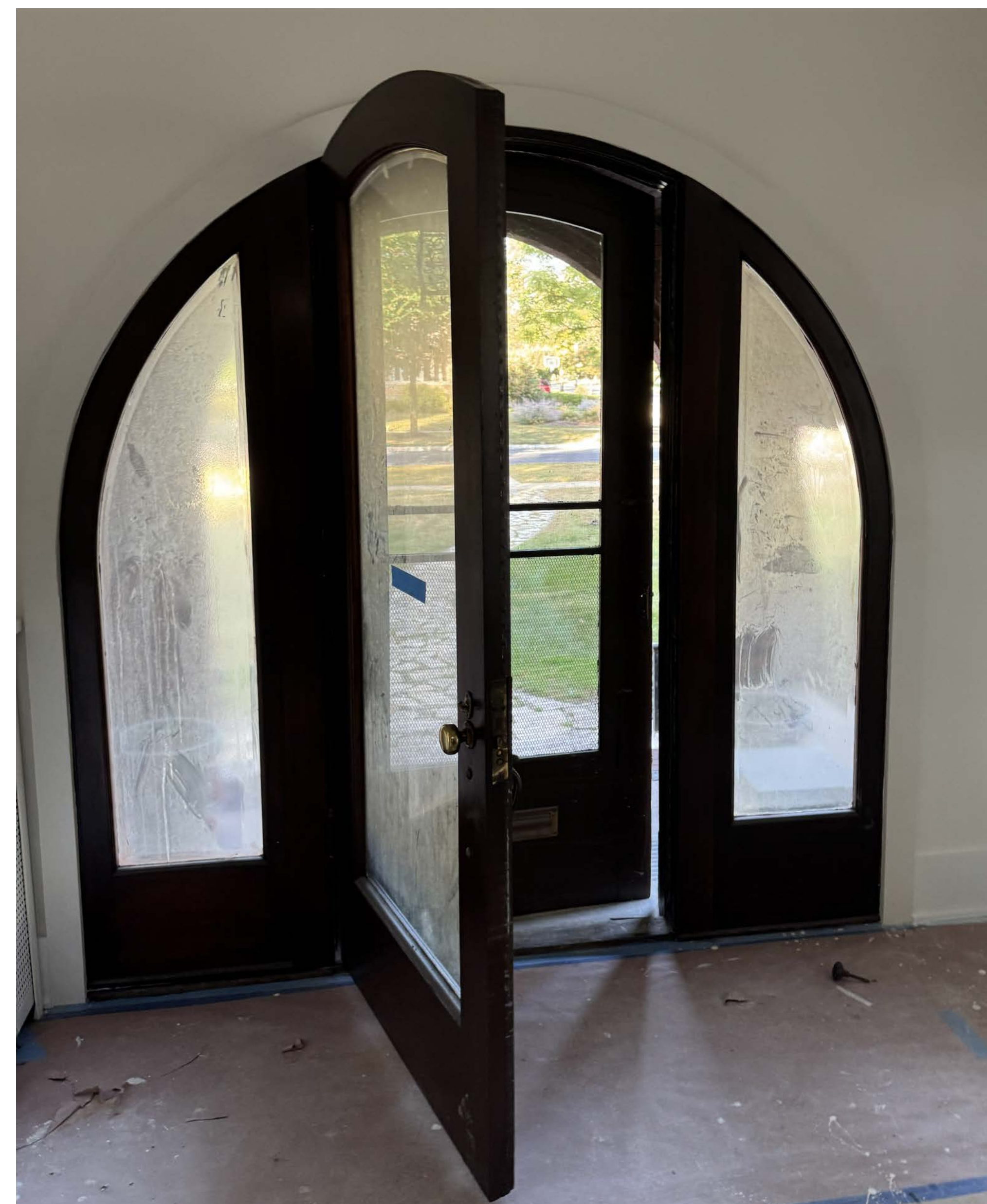
EXISTING FRONT DOOR
