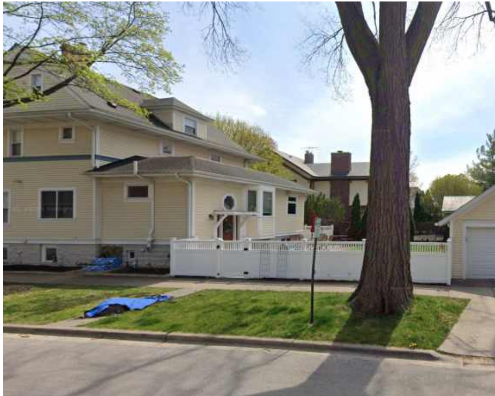
EXISTING REAR ELEVATION – FROM OAK STREET - NORTHWEST CORNER
