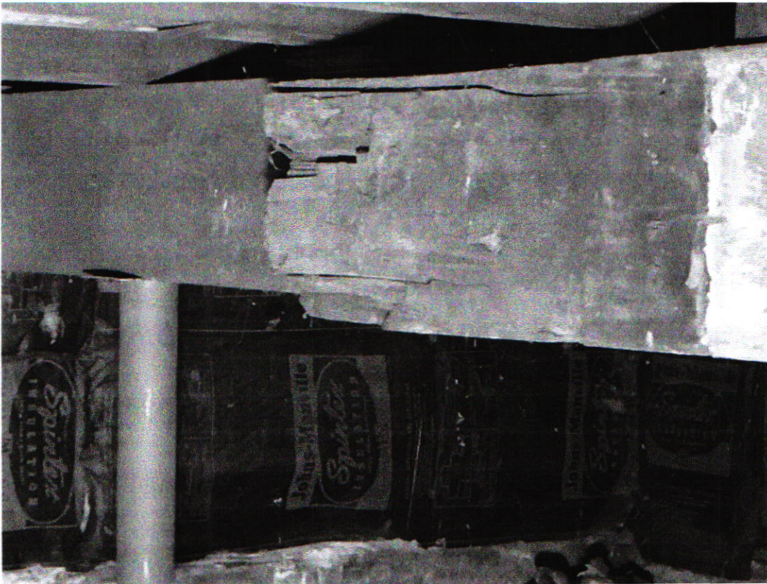
Photograph #6 - unsupported beam end under sun porch
