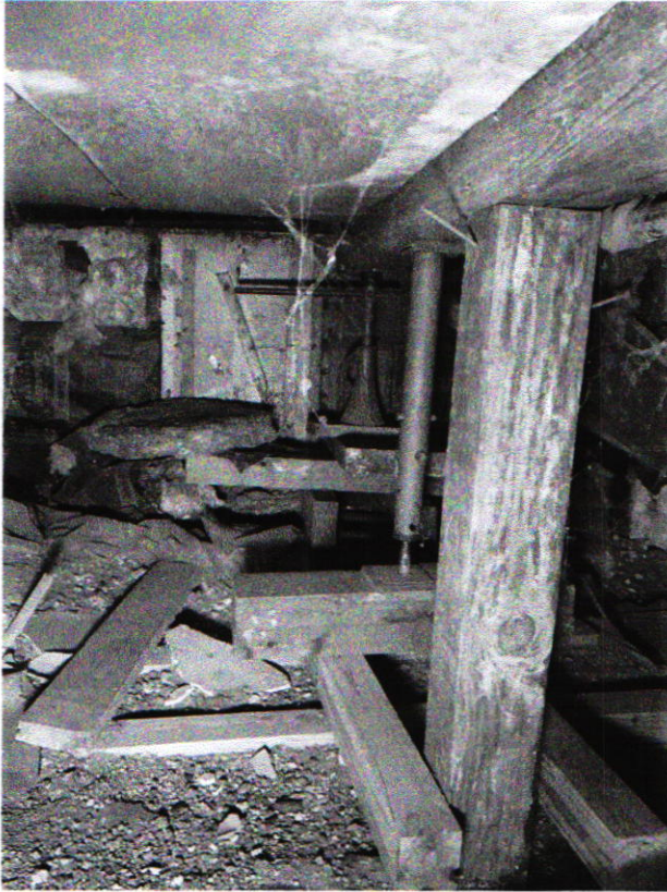
Photograph #7 - shoring & posts below southeast corner area
