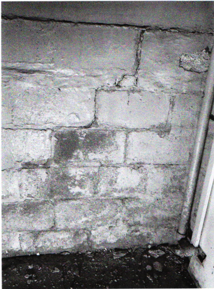
Photograph #2 - Foundation wall crack, southeast corner
