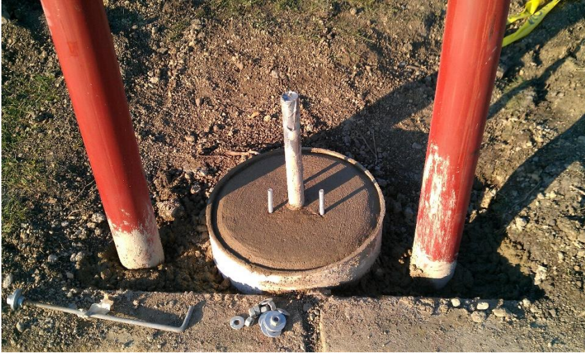
Figure 4: Typical Concrete Installation with Conduit and anchor bolts pre-set, protective bollards also installed.
