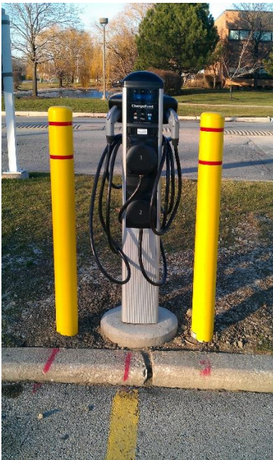
Figure 5: Example of Installation Completed (CT2021 Charger)
