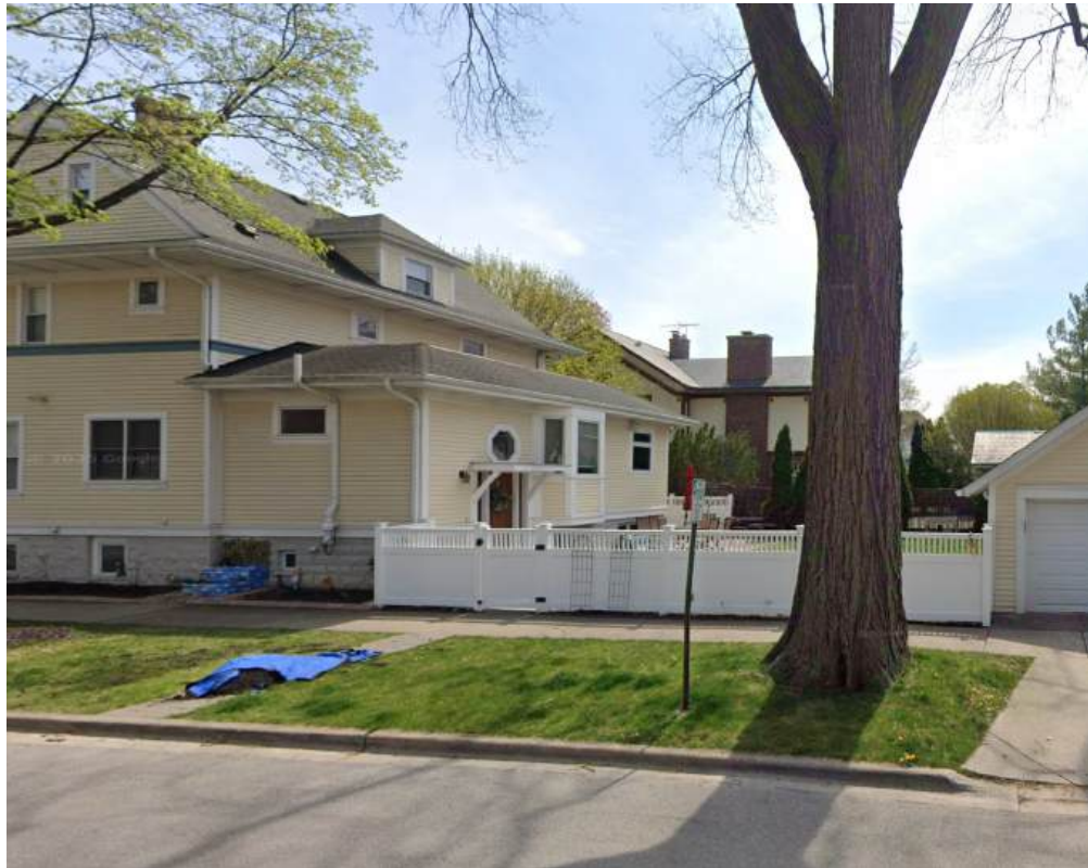
EXISTING REAR ELEVATION – FROM OAK STREET - NORTHWEST CORNER
