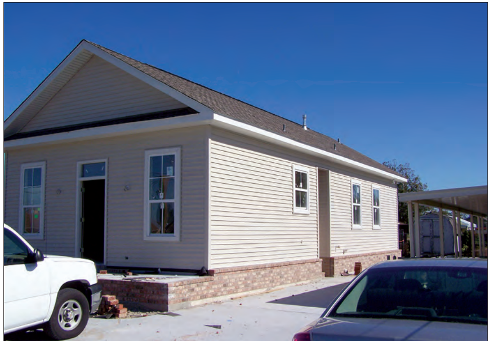
Figure 6-9. Typical mitigation reconstruction project.
