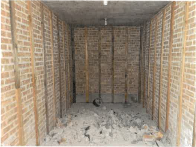
7618 W Madison River Forest, II Transite walls removed from vault
