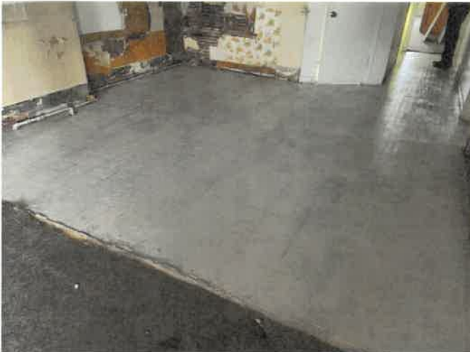
7612 W Madison River Forest, Il 2 nd floor vinyl flooring removed
