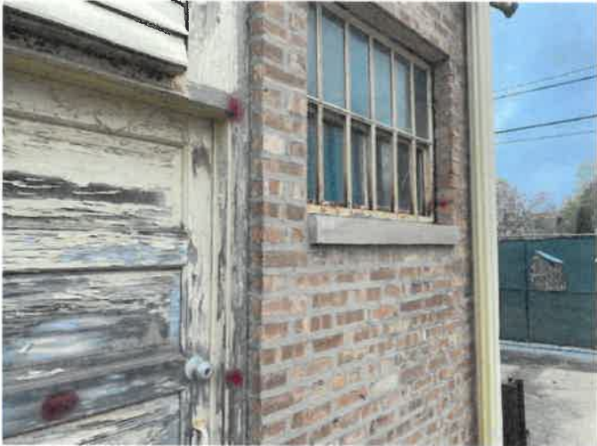
7618 W Madison River Forest, II Exterior door and window caulk removed
