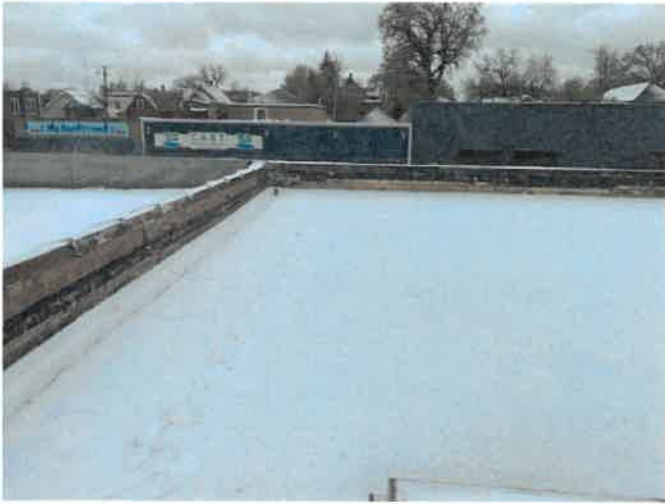
7618 W Madison River Forest, Il Exterior Roof Flashing removed
