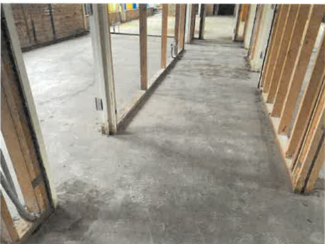
7620 W Madison River Forest, II Vinyl floor tiles and black mastic removed
