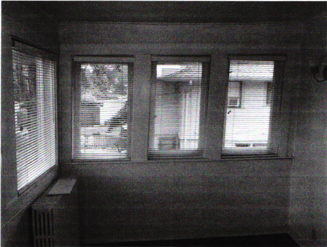
Photograph #9 - south exterior wall above shored area in southeast corner
