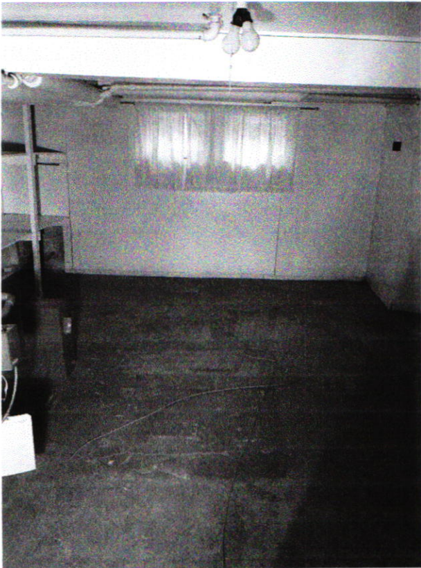
Photograph #4 - location where column removed. Pier visible in floor.
