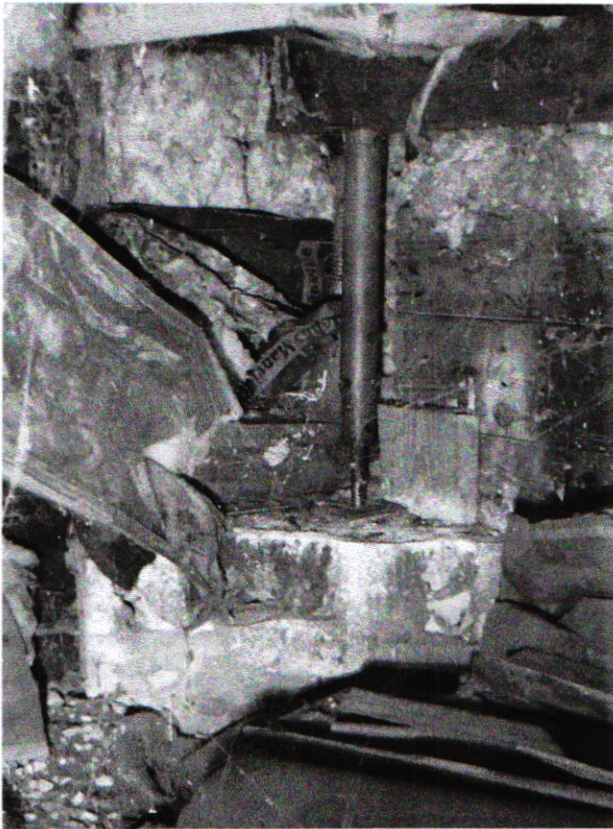
Photograph #8 - support at southeast corner of building
