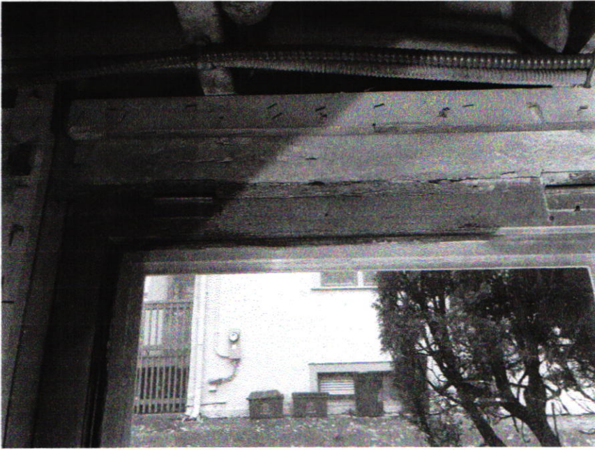
Photograph #1 - (2) flat 2 x 4's used as a header
