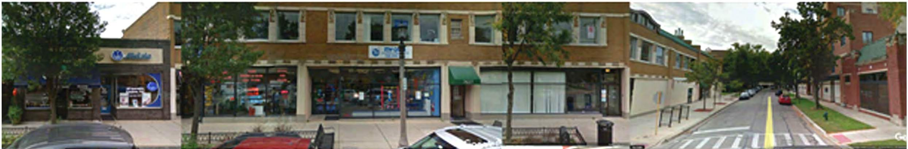
2- STORY COMMERCIAL BUILDING
