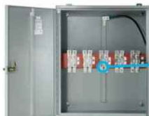
Generator lugs rated for Type W cable.
